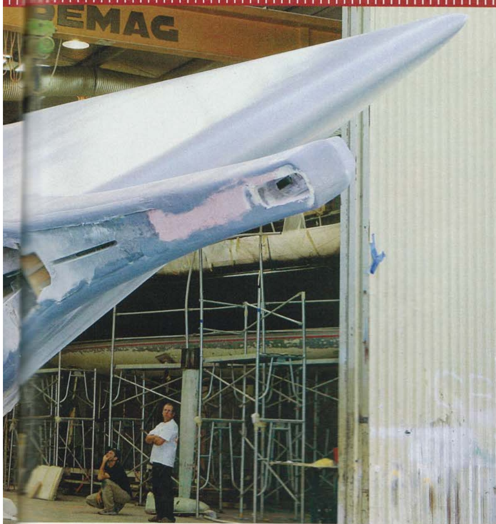
Wild Oats XI , a 98-foot Reichel/Pugh design, is rolled upright in the shop to allow builders to finish the cockpit (left) and interior. The boat was built in less than 10 months so it could compete in the '05 Rolex Sydney Hobart Race.
